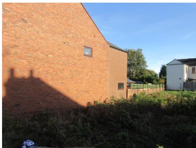
Photo of side elevation of No 65 St Johns Street
